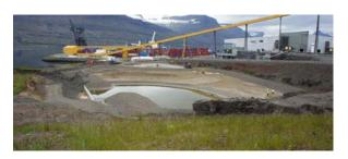
chemical and biological treatment. From the pre-treatment the stormwater is conveyed to a constructed wetland where a forebay removes solids and marshes to remove organic and inorganic contaminants. The wetlands were planted with vegetation indigenous to Iceland obtained from local farmers.
