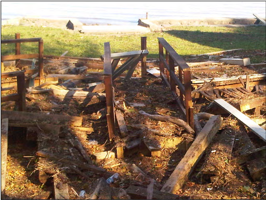
Photo 3. From Second Property North of Primary Residence Looking East: Substantial Portions of Dock Walking Surface Found.
