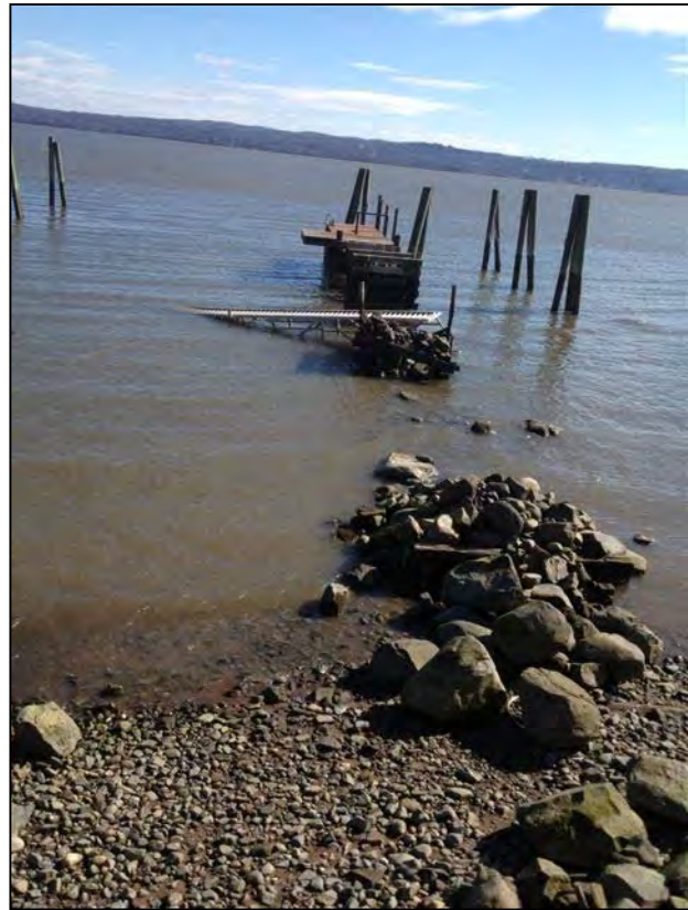
Photo 2. From Original Dock Location: Remnants of Primary Residence Dock Looking East.
