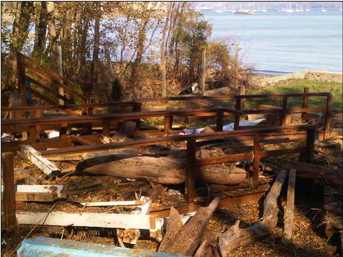
Photo 4. From Second Property North of Primary Residence Looking Northeast: Substantial Portions of Dock Walking Surface Found.
