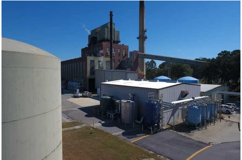
Gadsden Steam Plant. Link
